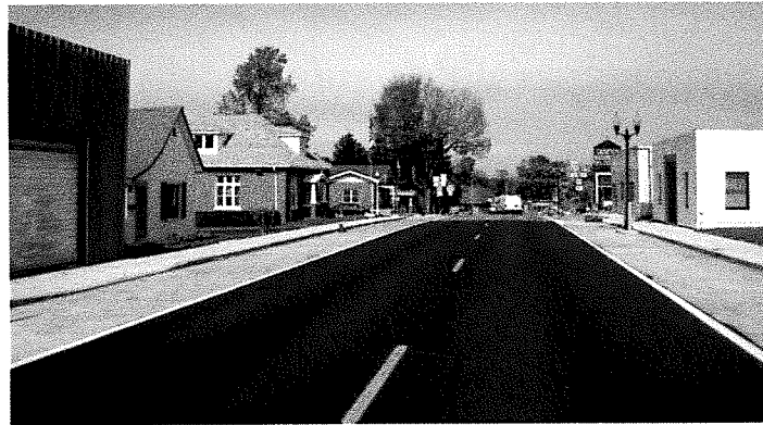
Hwy 8 Improvements - Desloge Drive - Federal Project No. STP-9900(073) City of Desloge
